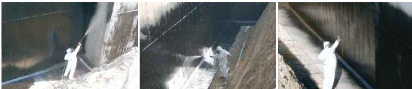
DERMARUBBER S/P : SPRAY ONTO THE FOUNDATION WALL
