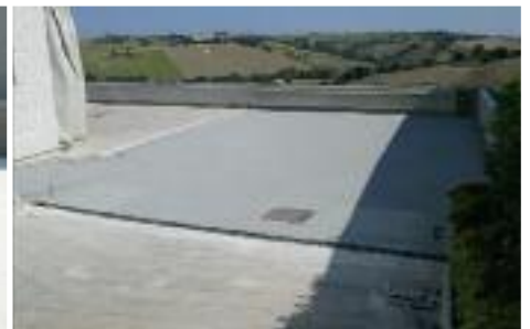
3. WORK COMPLETED WITH POLYTOP FINISH
