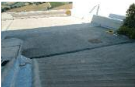
1. DRIVE-OVER DECK THAT IS WATERPROOFED WITHOUT DEMOLISHING
