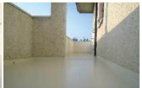
3. POLYTOP COLOURED FINISH / WORK COMPLETED
