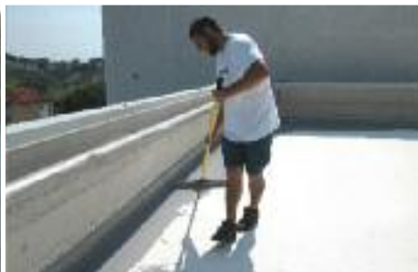
2. LAY THE DRIVE-OVER, SELF-LEVELLING WATERPROOF PRODUCT POLYROOF
