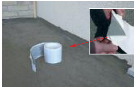
2. WATERPROOF JOINTS AND CONNECTIONS POINTS WITH CASABAND SA
