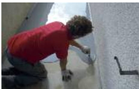
1. APPLY THE SELF-LEVELLING PRODUCT POLYROOF
