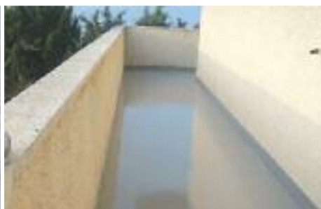
2. THE DECK IS READY FOR PAINTING
