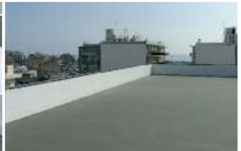
3. APPLY THE LAST COATING OF DERMACEM / WORK COMPLETED YOU MAY: A) TILE THE SURFACE B) COAT THE SURFACE WITH ACRYTOP
